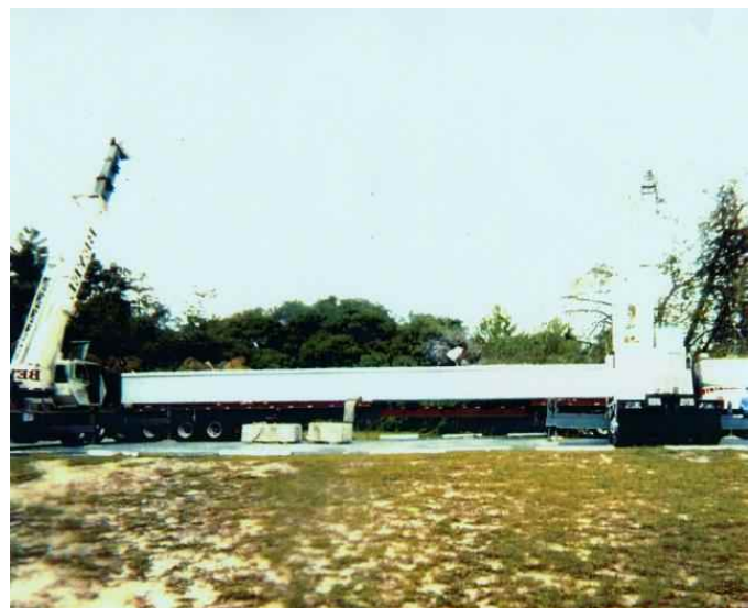
Figure 18. Photo of 72 Foot Long Monorail Guideway Beam Delivered to Maglev 2000 Facility in Florida from Fabrication Site in New Jersey
