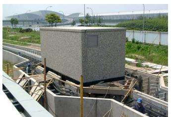
Figure 2: Switch station and cable tray on the Shanghai track
