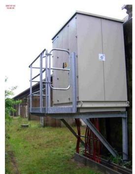
Figure 3: Compact switch station mounted at a guideway column
