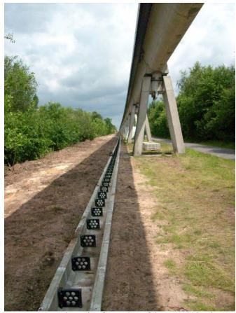
Figure 5: TVE track section for testing of the new cable clamps
