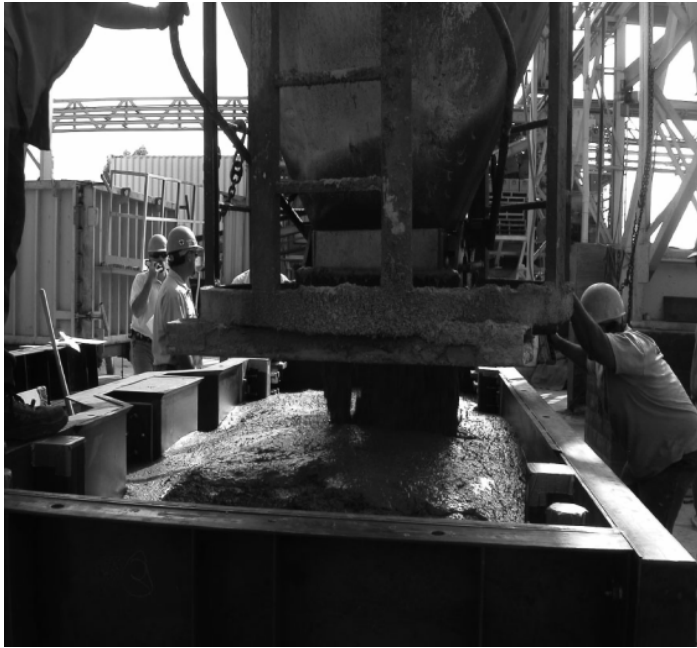
Figure 2: Fiber concrete poured into forms
