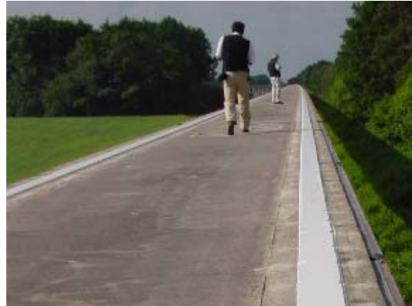
Fig. 5 Coated guideway for the qualification tests.
